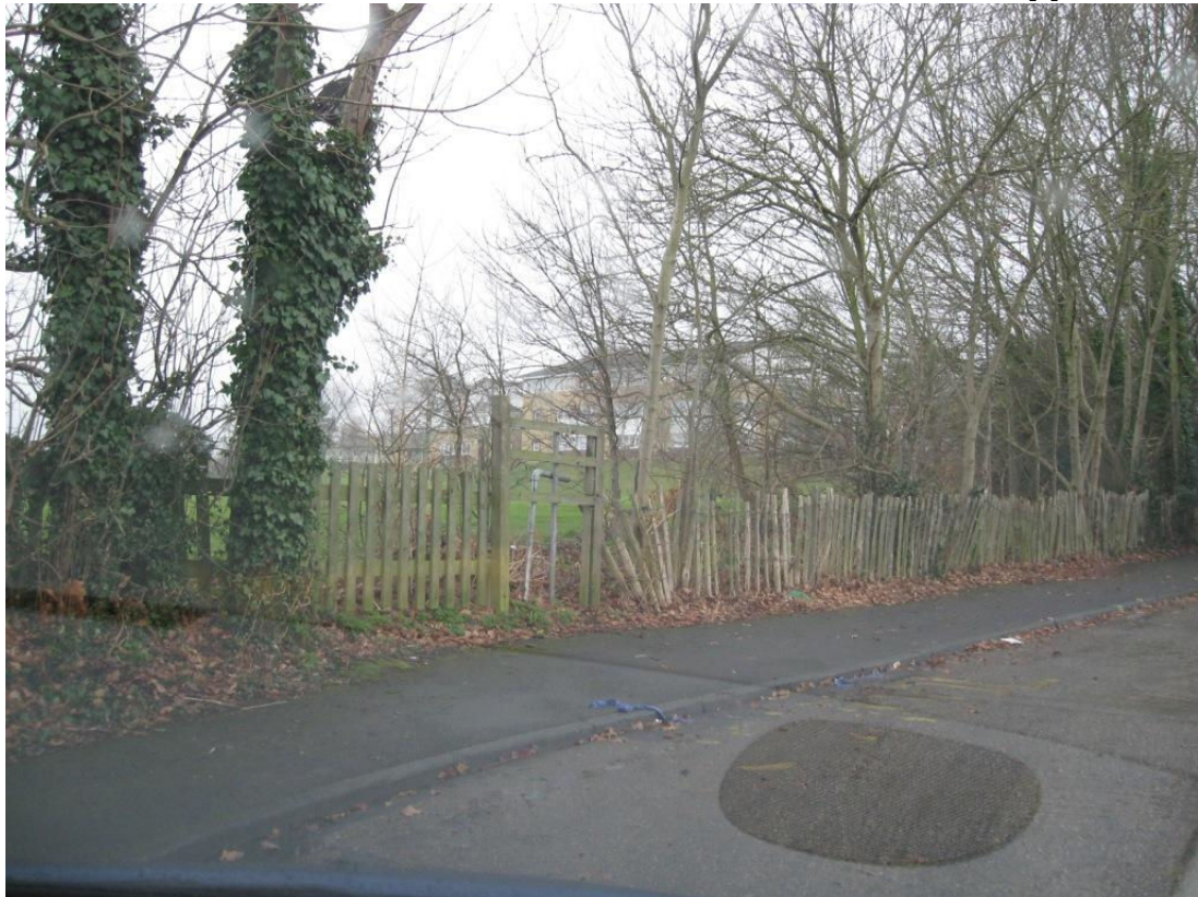
View looking west at bus lay-by
